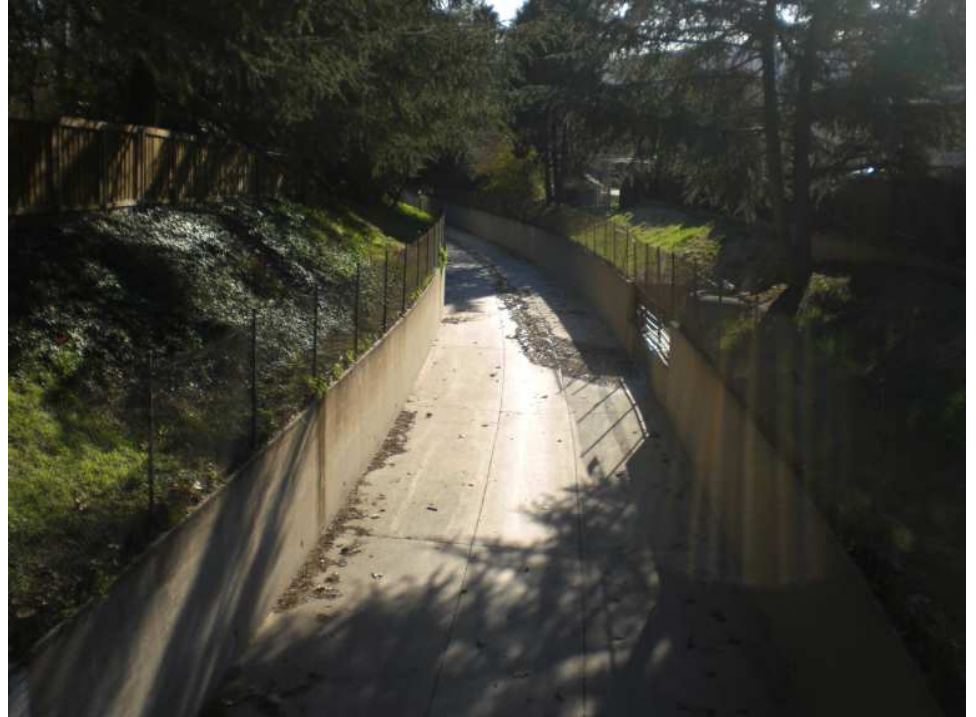
Halls Canyon Creek at Cross St. (facing downstream). The channel begins from Halls Debris Basin and drains to Verdugo Debris Basin.
