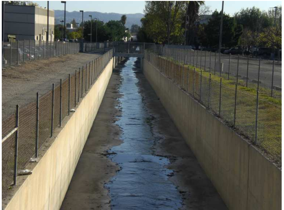
Limekiln Canyon Wash at Plummer St. (downstream). The channel begins at Limekiln Debris Basin and drains to Wilbur Debris Basin.
