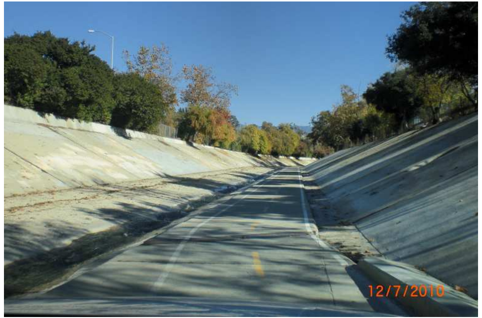
Arroyo Seco Reach 1 with a bike path next to a low flow (downstream). The 7-mile reach begins at Holly St. in Pasadena as a rectangular channel for 2 miles and transition to trapezoidal from San Pazqual Ave. to its confluence with Los Angeles River Reach 2.
